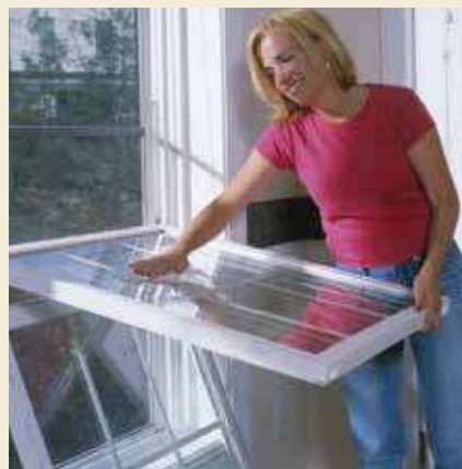
Tilt-in top and bottom sash for easy cleaning.
